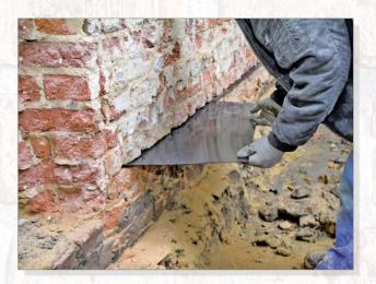
Finally fastening the cut joint with static load bearing plastic wedge plates, at a distance of maximum 25 cm over the entire wall cross section (load bearing capacity minimum 500 kp/cm2).
