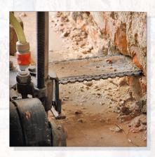
2. Sectional removal of the wall work with PRINZ chainsaw PMS 60, PMS 25 or EED 3.5 for brick walls similarly removal with PRINZ diamond rope saw PDSS 500 for rubble stone or mixed walls. Thus, the length of cut of up to 1,00 m is suited to the constructional and static conditions present.
